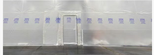
Pocket Doors are a perfect solution for when personnel need to enter and exit containment areas regularly.
